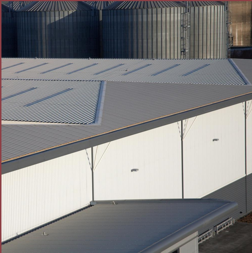
Trapezoidal Insulated Roof Panel KS1000 RW
